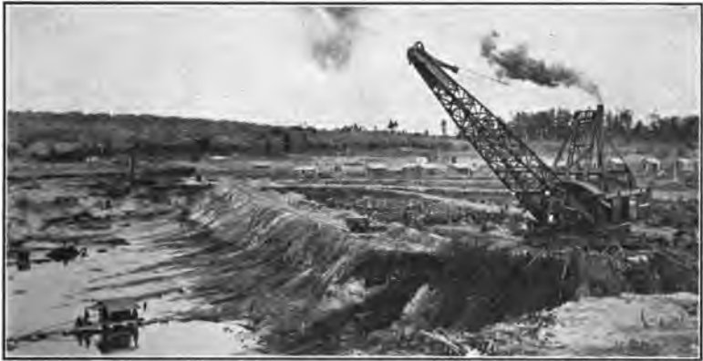
BALKAN MINE—JULY 1, 1914. VIEW LOOKING SOUTHEAST, SHOWING SOUTH HALF OF CUT.
